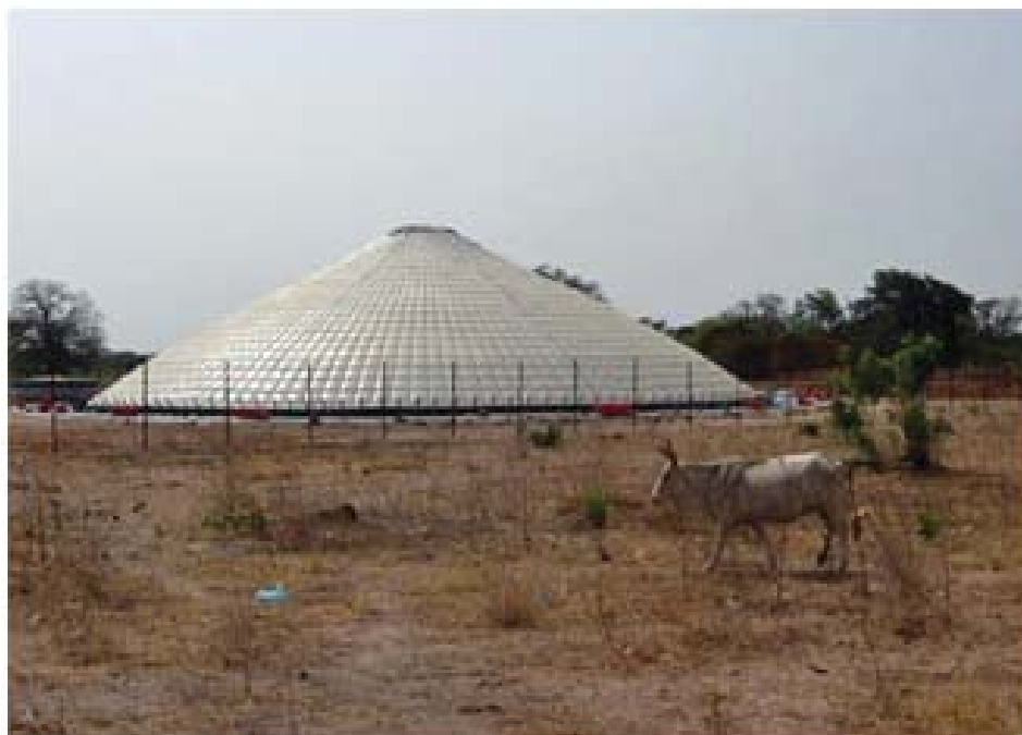
Figure 3: Huge Dutch water pyramid on the Indonesian island Pomana produces around 1000 liters (about 260 U.S. gallons) of clean water per day.
