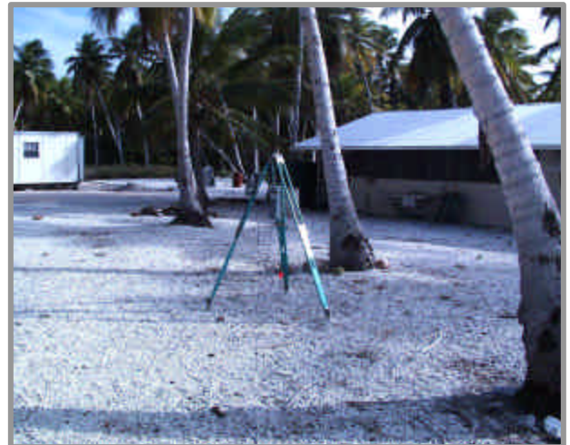
Lack of coral fill in the area surrounding original construction camp.
