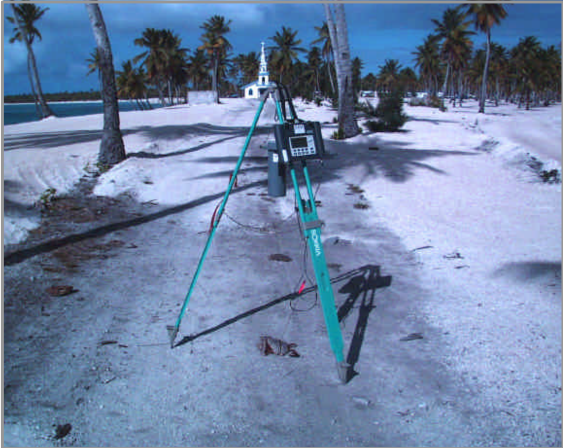
Unscrapped road surfaces
