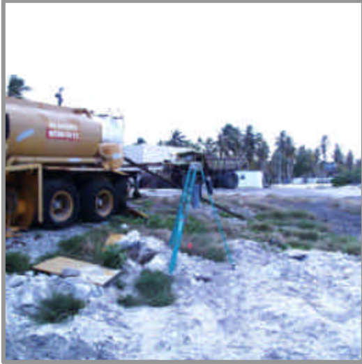
Unscrapped areas and dark colored fill around generator building.
