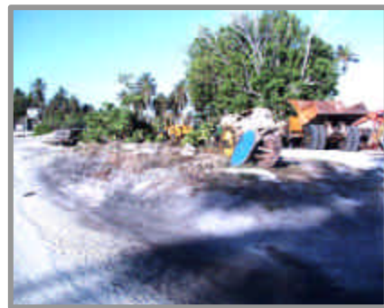
Unscrapped surfaces adjacent traffic area
