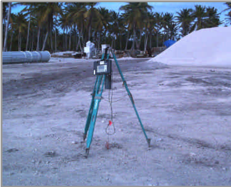
Figure A-6. Beach frontage N-W of service area and adjacent asphalt plant.
